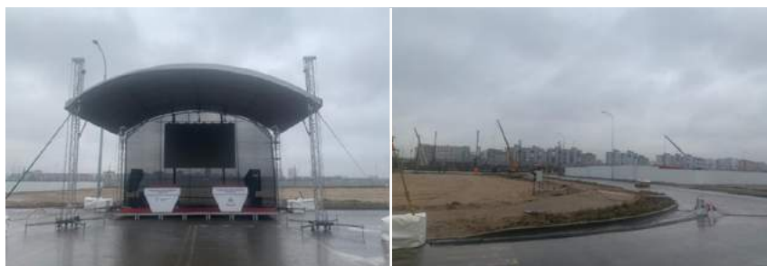
Construction of cultural cluster objects, Kaliningrad, February 25. Photo by Katerina Novikova
