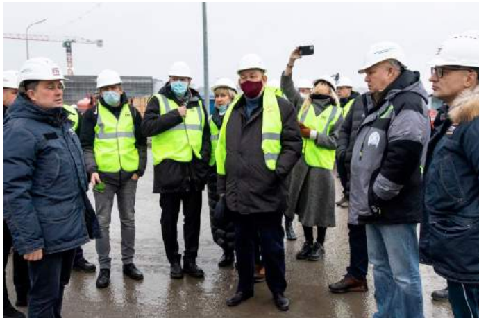
Vladimir Urin visited the construction site of the Bolshoi Theatre branch in Kaliningrad. Photo:Yulia Vlasova
