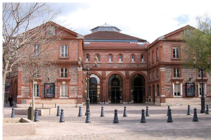
Halle Aux Grains in Toulouse. Photo / gps
